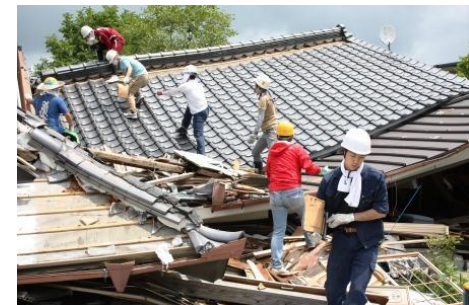
Volunteer activities at the areas damaged by the Kumamoto Earthquakes
