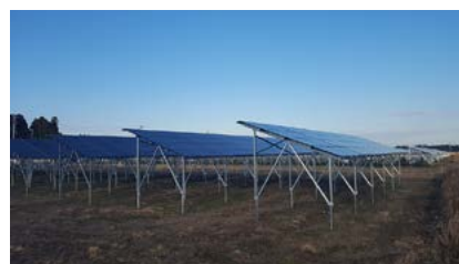
Solar panels attached to pillars built on farmland by Toyo Energy Farm Co., Ltd.
