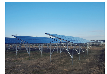
Solar panels mounted on a framework above farmland (Toyo Energy Farm Co., Ltd.)
